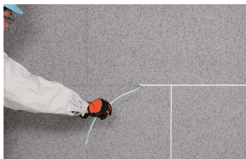
Removing groove lines.
